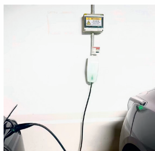
Installed the pure electric vehicle charging piles
